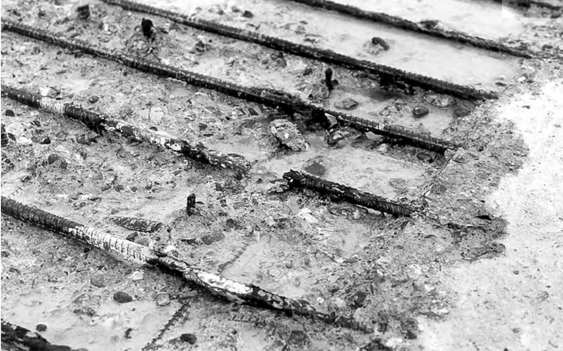
Figure 1. Corroded carbon steel reinforcing bar in elevated roadway of Gardner Expressway, Toronto, Canada
